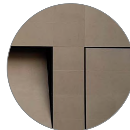
Particolare porta filo muro Detail of the door flush with the wall
